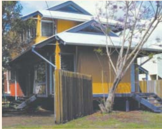
This energy efficient award winning house, designed by Paul Trotter, uses good design (including large overhangs and louvres) to combat the solar overheating problems presented by an east-west aspect. Provision of separate summer and winter living spaces allows comfort conditions to be optimised for best seasonal performance. All this was achieved with a lightweight timber structure.
