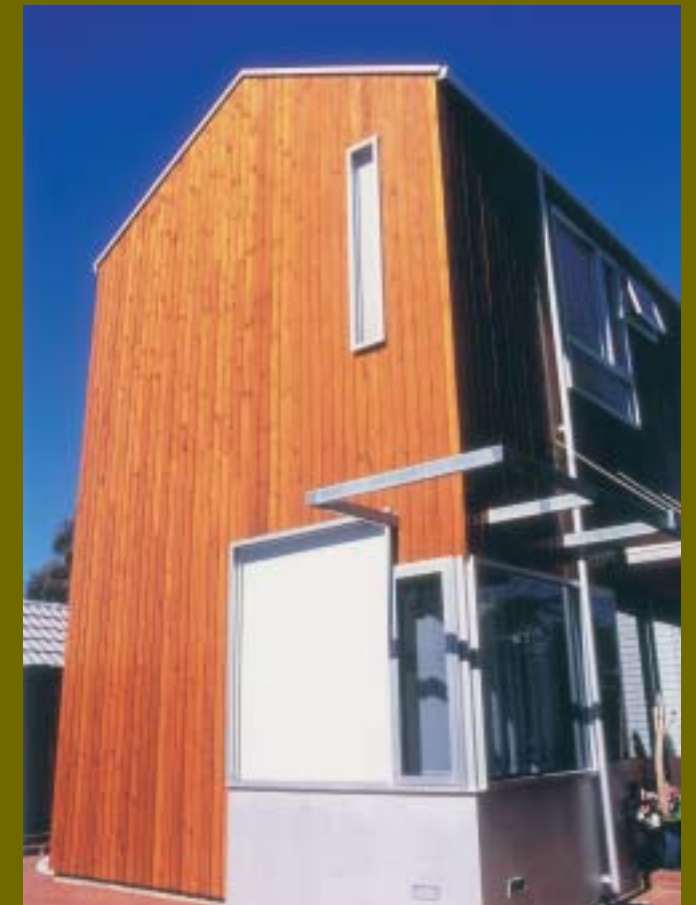
The striking extension to the 80 year-old workers' cottage that features WESPINE structural framing.
